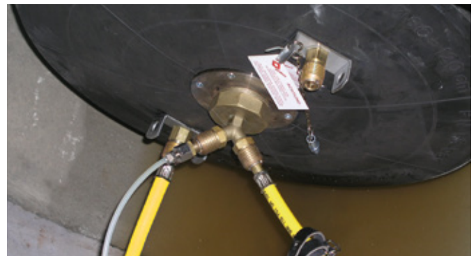
Air pressure test
